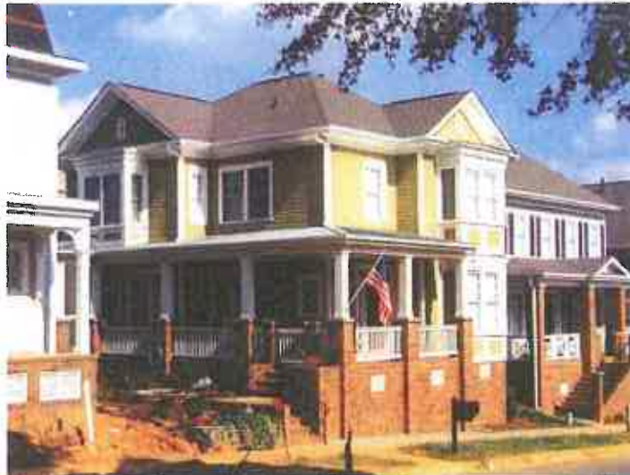
This residence is articulated on all sides with windows, wrap around porch, variances in façade depth and color and material changes.
